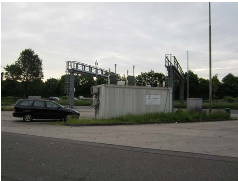
Figure 16: Field test site Bornheim, motorway parking lot
