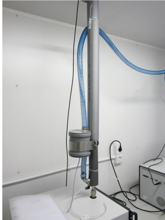
Figure 4: Active ventilation of the sampling system used for field testing
