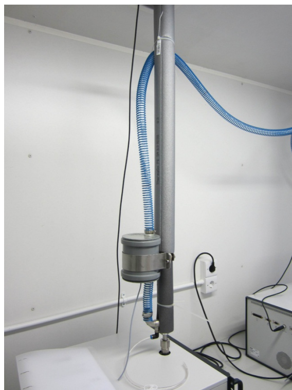
Figure 4: Active ventilation of the sampling system during field test
