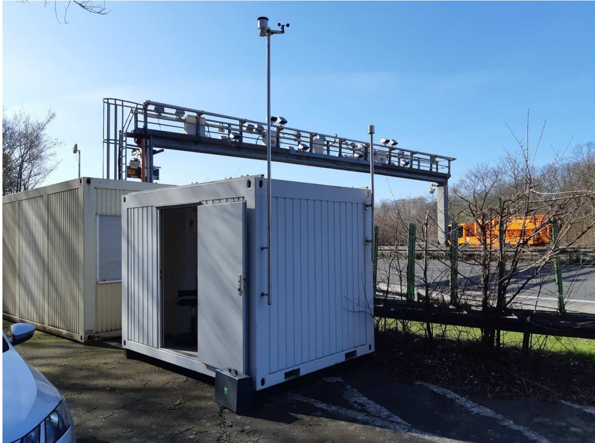
Figure 8: Measuring station for conducting the field test
