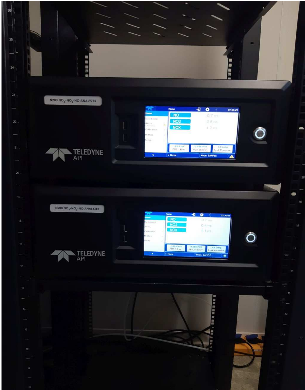
Figure 9: N200 in the measuring station during the field test
