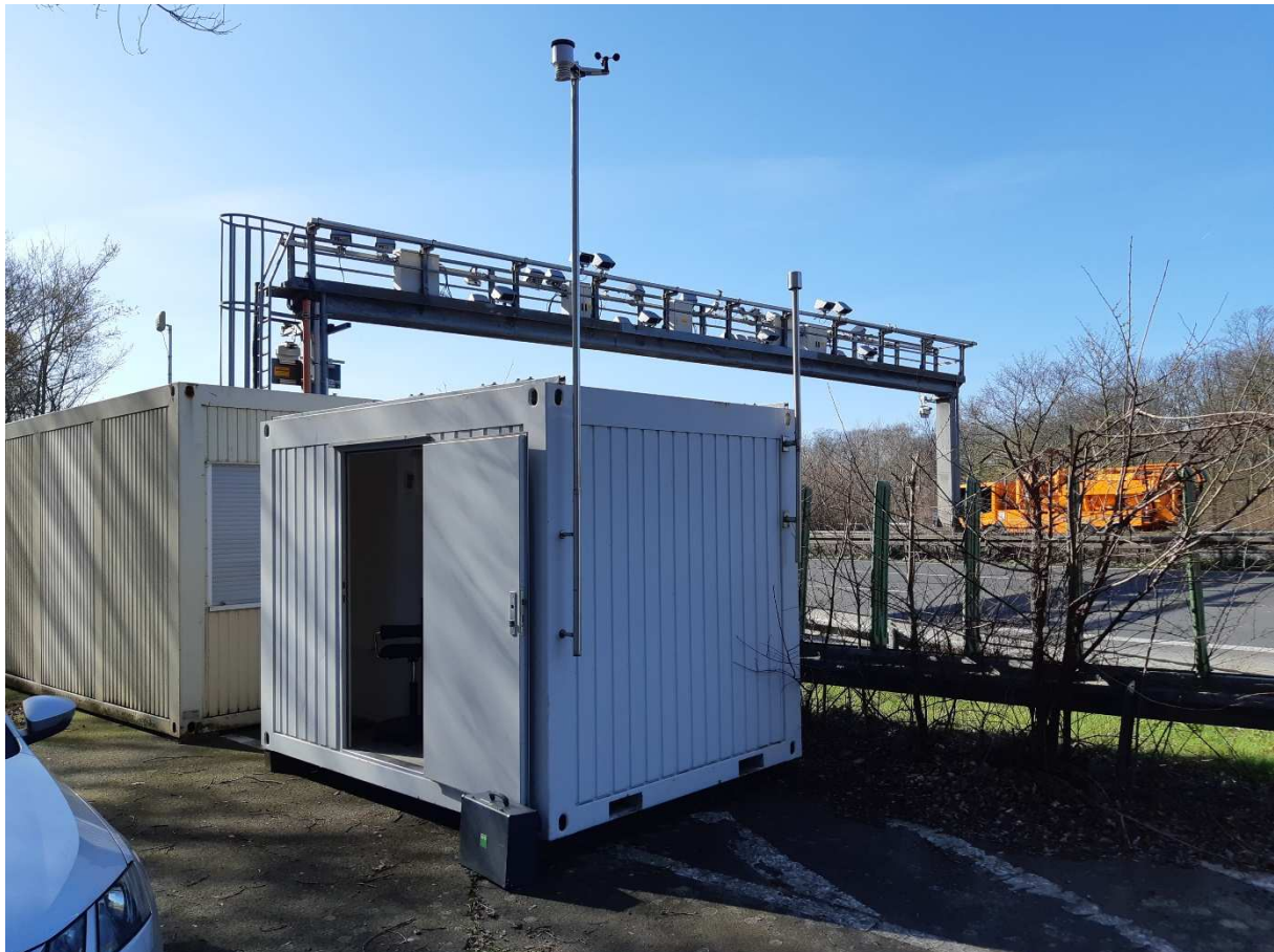
Figure 8: Measuring station for conducting the field test
