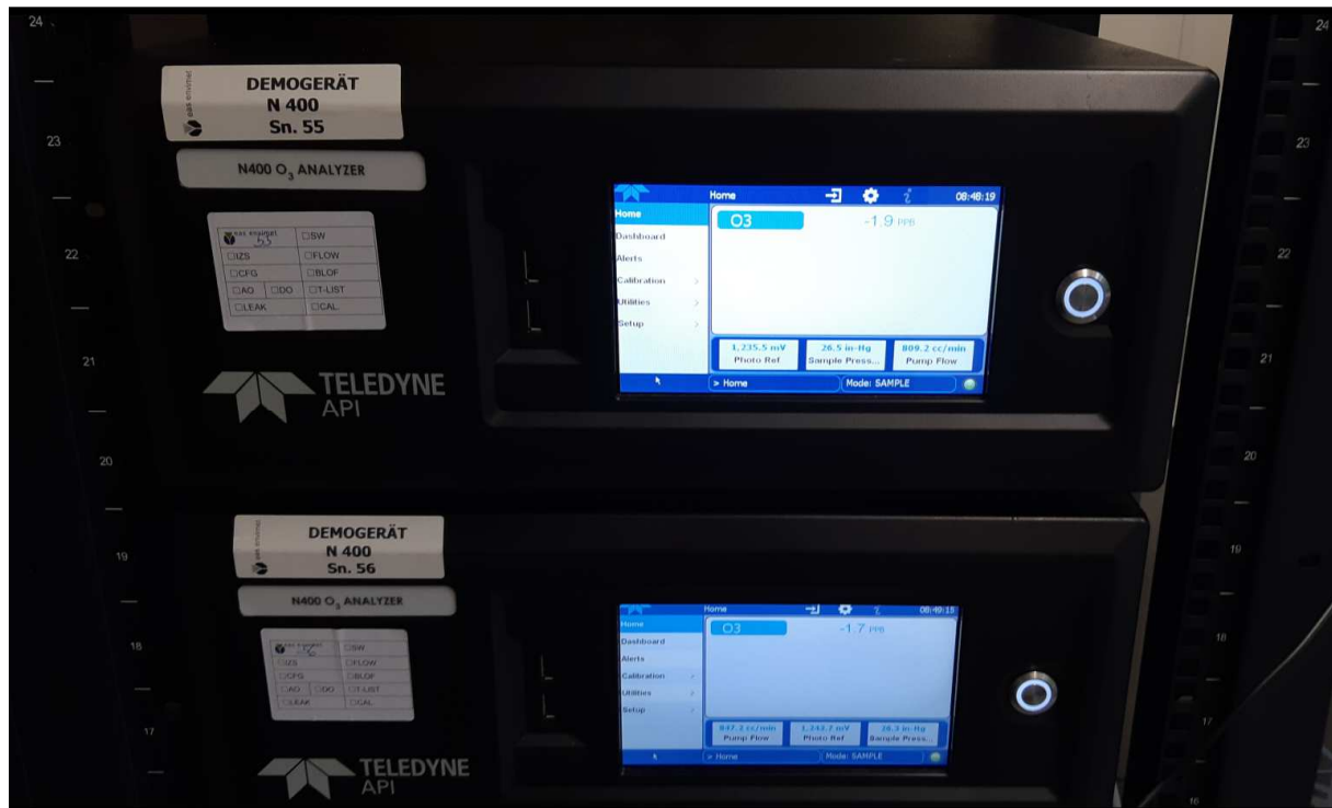
Figure 8: N400 in the measuring station during the field test
